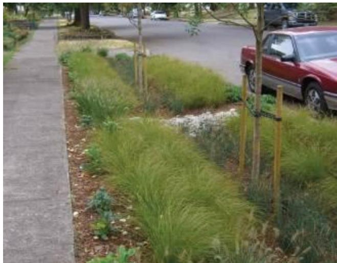
Example of a retrofitted planting strip designed to treat stormwater runoff from the sidewalk and street. Source: Green Streets Fact Sheet, Portland, Oregon.
