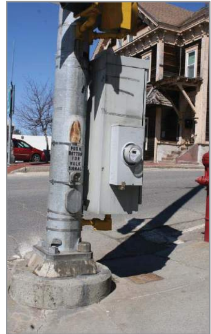
A utility pole and transformer box obstructs the crossing area and curb-ramp on North Main Street.
